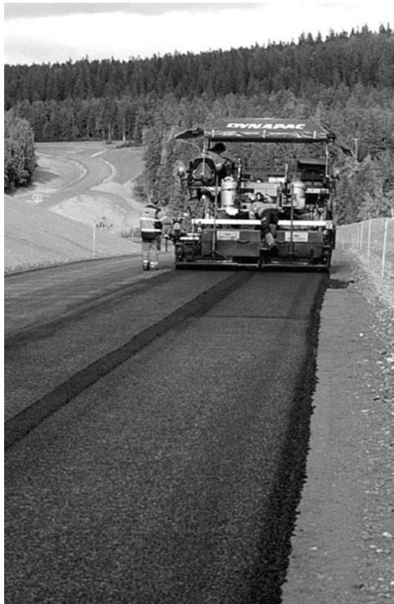
FIGURE 11.12 Paving of semi-dense cold mix asphalt.
