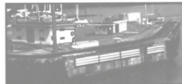
SOLIDUR fender facing in canal system.
